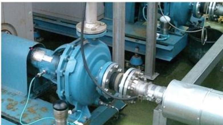
BE Bently Nevada vibration energy-harvester-powered wireless sensor node installed for machinery condition monitoring at Shell's Nyhamna Gas plant.
