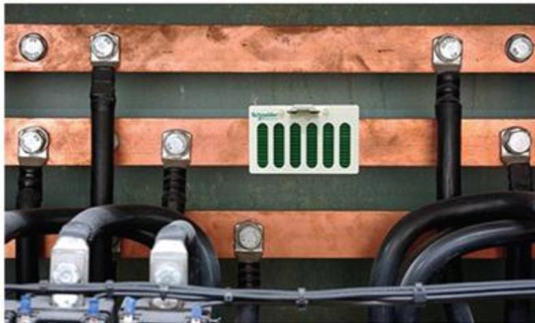
Temperature monitoring WSN powered by Micropelt's thermal harvester.
